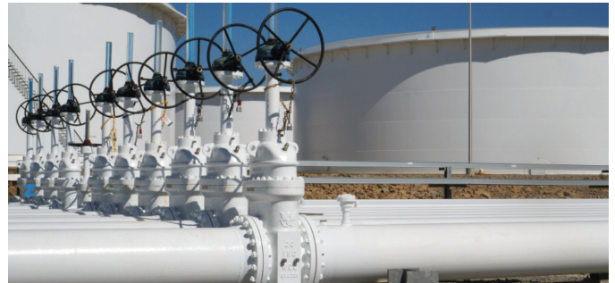
20" CL150 Slab Gates installed at Oklahoma Facility
