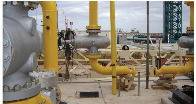
Expanding Gate Valve Installation
